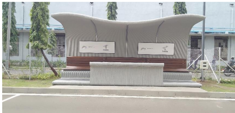
Proof Of Concept using 3DCP technology to create a sustainable and inclusive bus shelter
