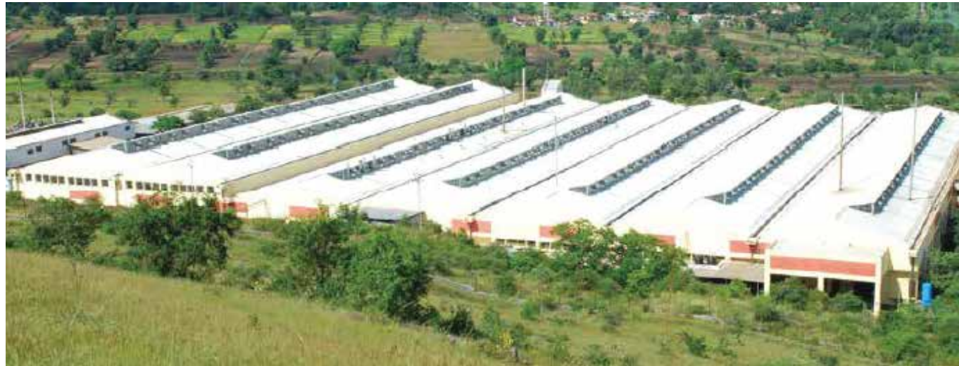
Aerial View Of The Godrej Air Conditioner Manufacturing Facility, Shirwal, Maharashtra
